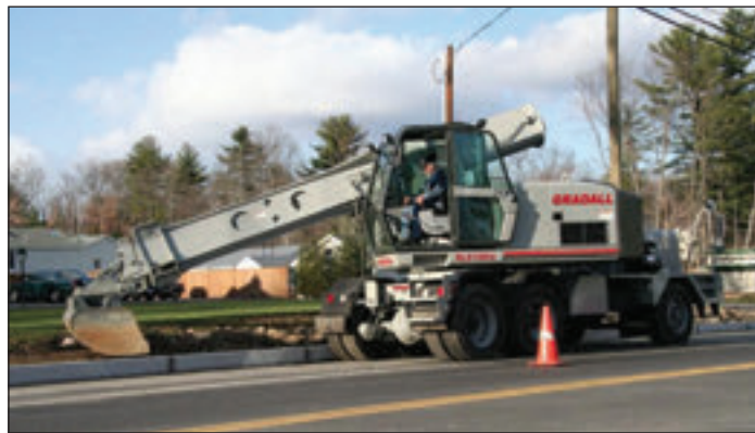
Pictured from top: Two FWF Gradall machines at work removing the worn road surface of a city street in Shaker Heights in 1945. The Swetland building at 26011 Chagrin Blvd. with a Beachwood Police Dept. patrol car in 1938. The Gradall Model XL5100 III being used in the finish grading of the devil-strip along the side of a new city street.
