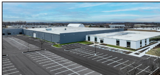
An aerial view of the Commerce Park project site.
